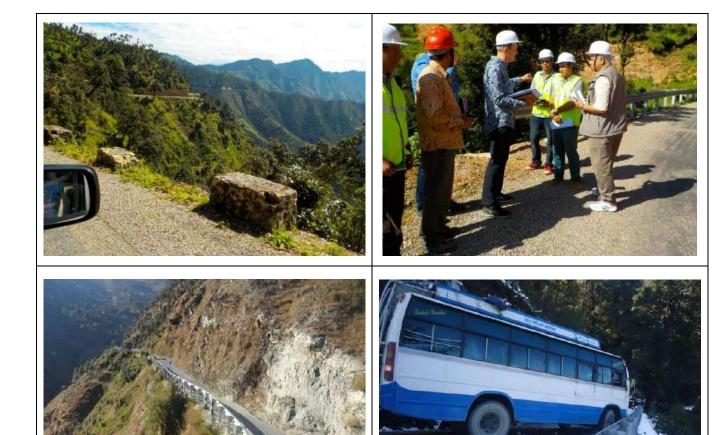
**Figure 4.4: Roadside Barriers in Nepal**. The GRSF funded construction of roadside barriers on cliff-side roads in Nepal, showing in order the road without barriers, during construction, at completion, as well as an example of a bus which was prevented from going over the cliff by the barrier
